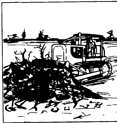
Brush Clearing: Lower blade a few inches into the ground and move forward Lift blade when brush is out to loosen earth from roots.
